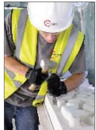
*Man at work! A mason cutting a new vermiculated panel.*
