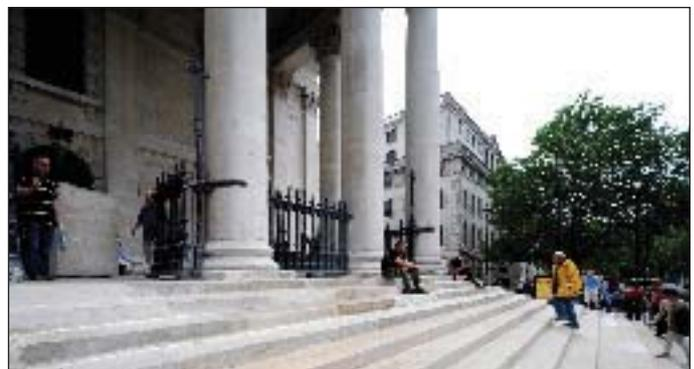
*The famous steps leading to St Martin's main entrance inside the west portico. Most of the steps were turned over and refaced rather than replaced with new stone.*
