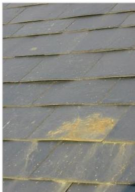
The effect of a pyrite dissolving and leaching to cause runs of discolouration on a roof.
