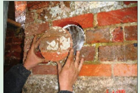
*Going, going, gone! Plugging the Cintec anchor bores with a disc cut from the end of the core removed.*
